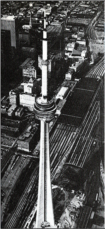
Slipformed and post-tensioned, the CN (Canadian National) Tower, Toronto, Ontario, is world's tallest freestanding structure at 1805 feet. (49)
